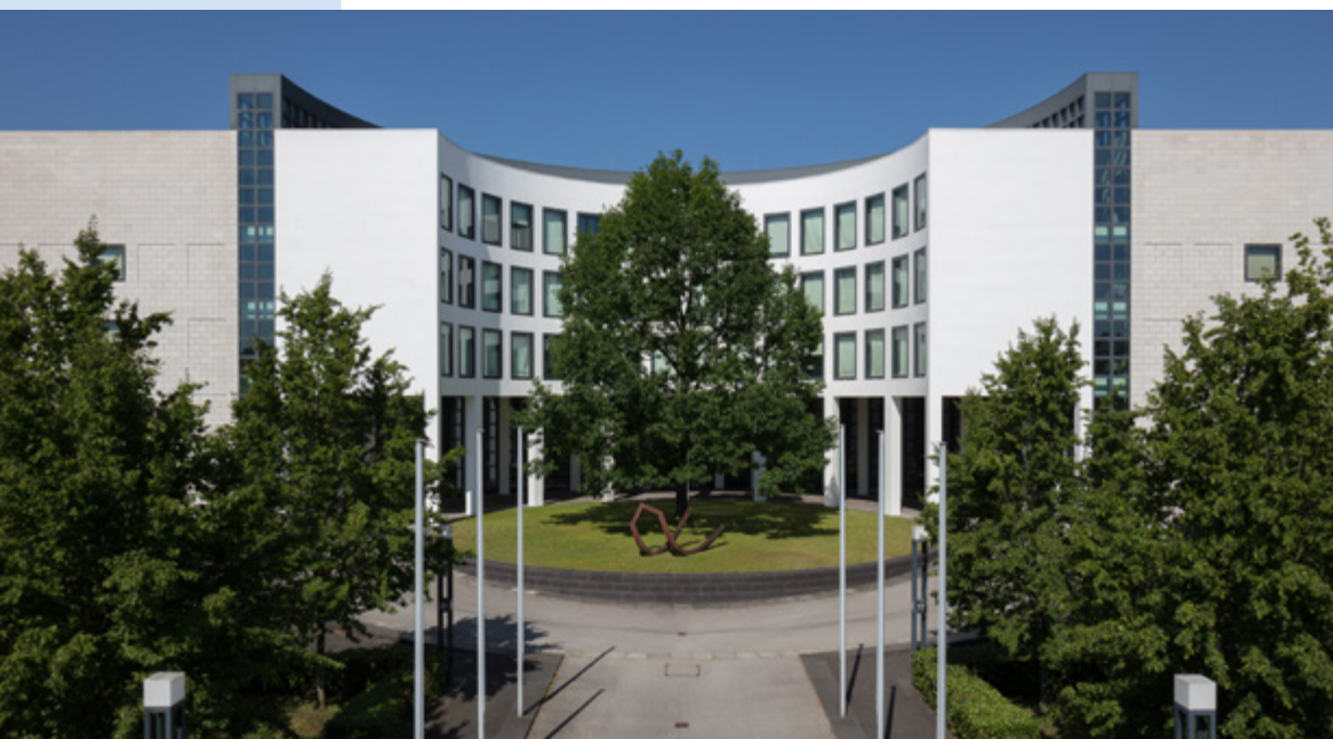
The Federal Public Prosecution Office building in Karlsruhe.
